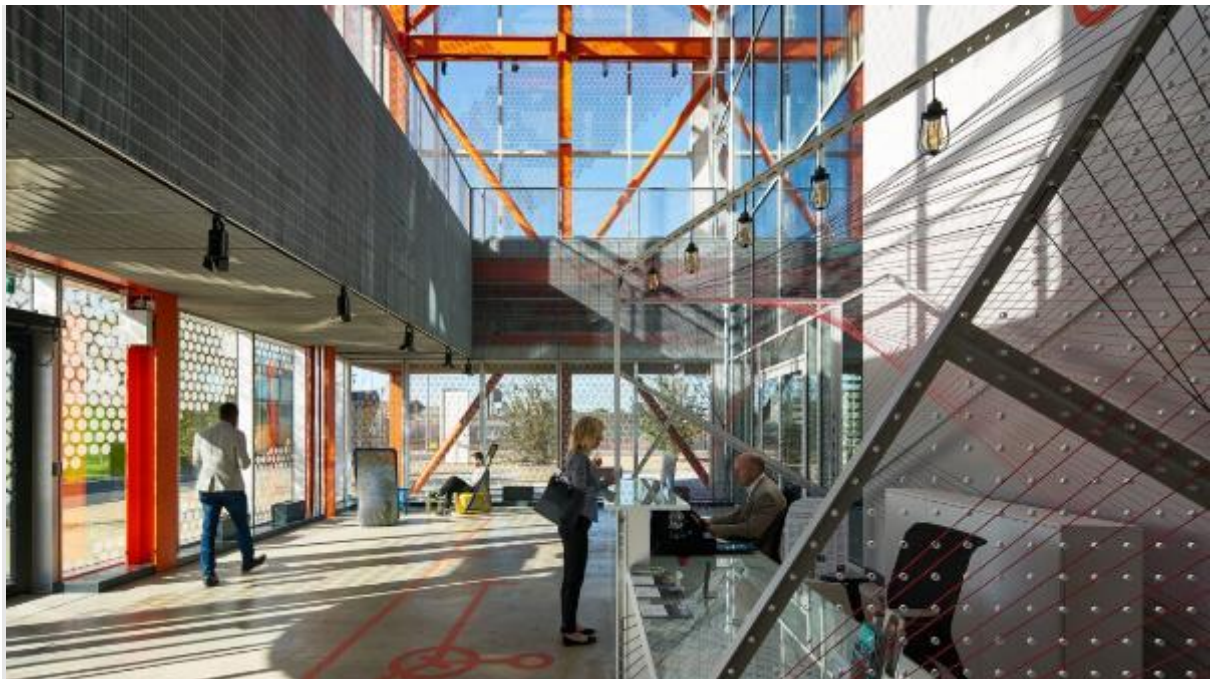
Figure 49 - Here East, Stratford: The refit of the London 2012 Media Centre into commercial space for creative and digital industries was inspired by the light industrial factories and yards of neighbouring Hackney Wick. The aim was to make a series of huge buildings more social, dynamic and flexible with the potential to evolve. The original windowless facade was removed to create a glazed outer layer of flexible work, studio and commercial spaces around the perimeter - maximising natural daylight, ventilation and views. Education, employment and enterprise coexist behind colourful animated facades featuring projecting/inset balconies with bright orange metalwork, brise soleil, and solar dot patterned glazing. The combination of elements is effective in breaking down the scale of the building.
