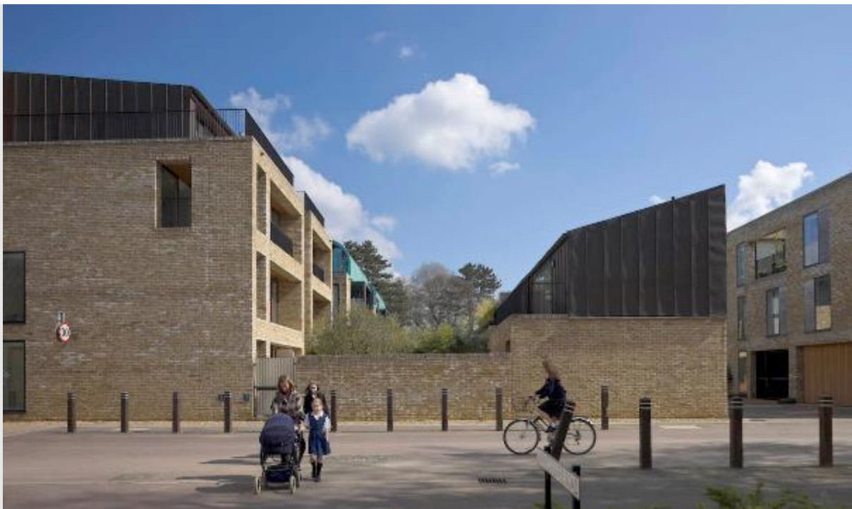
Figure 27 - Accordia, Cambridge: Adapting a traditional housing typology with a distinctive asymmetrical roof form, optimising light, ventilation, and internal connectivity whilst maintaining a terrace-like urban form to the street.
