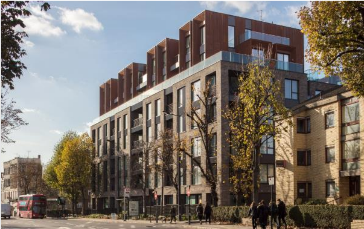
Figure 14 - Camden Courtyards, Camden: The scale and massing is moderated to respond to the surrounding townscape and broken down through materiality and detailing which reflects the industrial heritage of the site. The scheme achieves high density with a maximum height of seven storeys.
