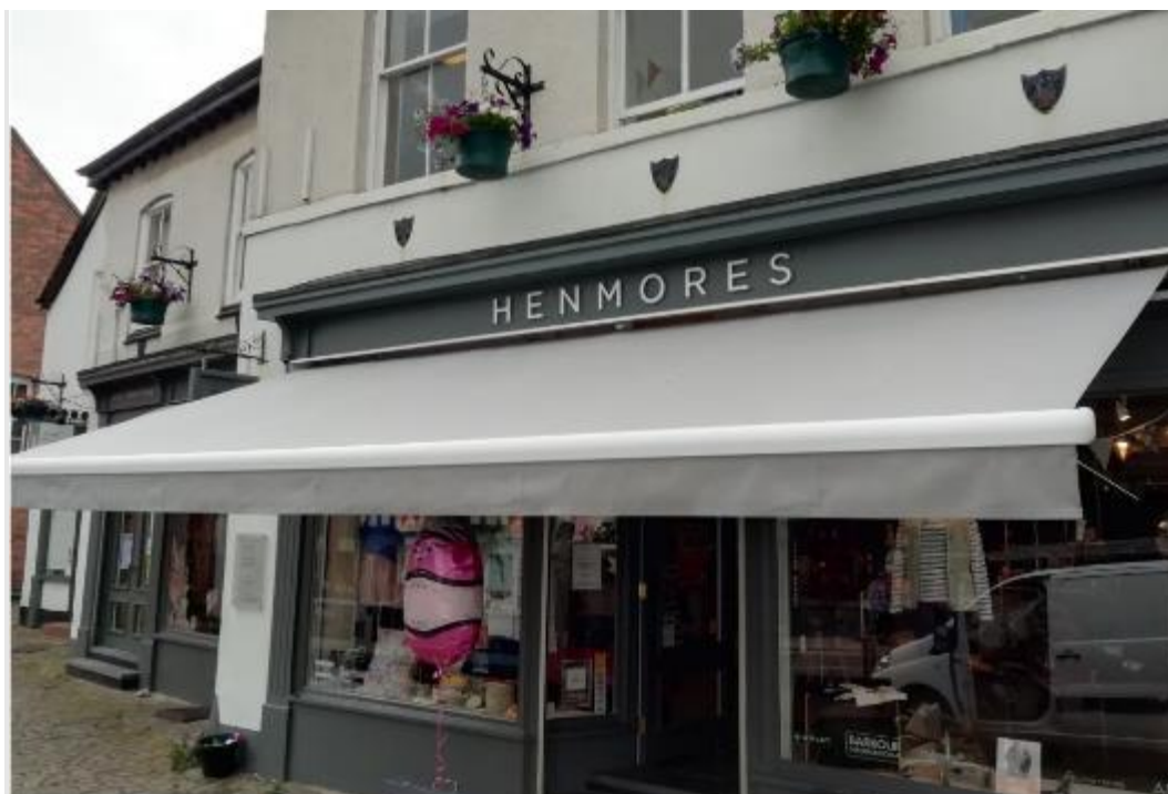
Figure 60 - A fully integrated retractable canvas canopy
