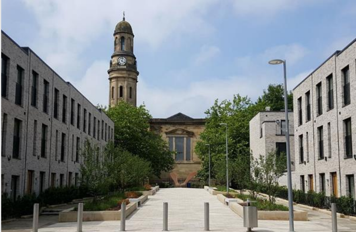
Figure 7 - Timekeepers Square, Salford: Reintroduces the historic street pattern of the area, while responding to the height, massing and rhythm of existing Georgian terraces. The new housing creates a positive setting for several Grade II listed buildings.
