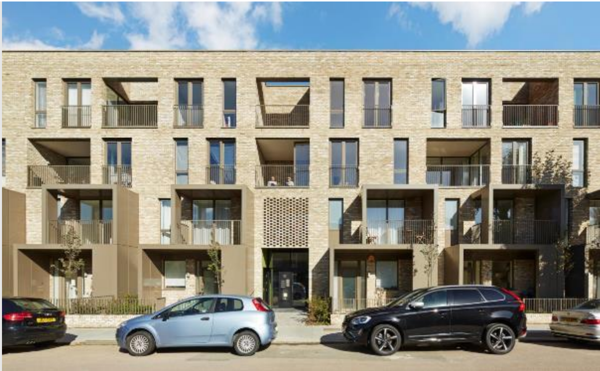
Figure 32 - Ely Court, Brent: A rhythmic composition of recessed windows, front porticoes, upper porticos and recessed balconies creates a highly articulated street facade.
