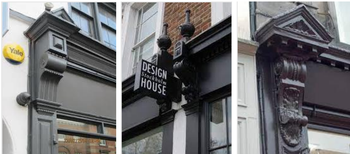
Figure 55 - Examples of decorative corbels which feature on traditional shopfronts
