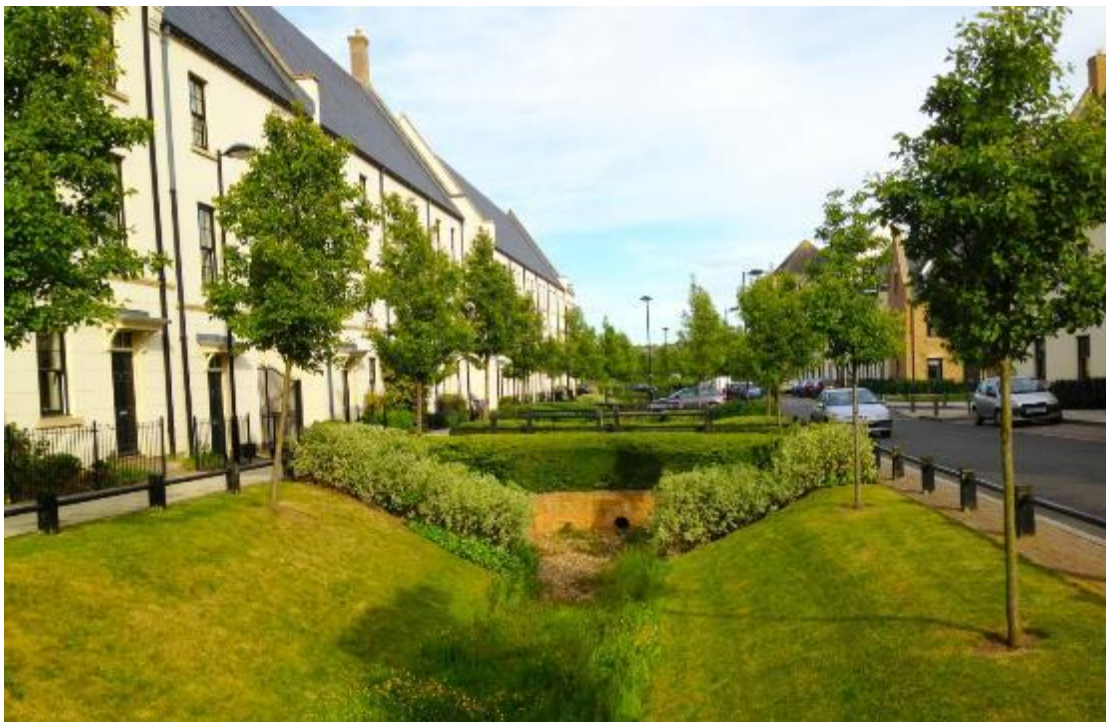
Figure 95 - Upton, Northampton: Sustainable Urban Drainage Systems are incorporated throughout the masterplan (an urban extension of approximately 1350 homes) with generously sized swales contributing to the character, identity and biodiversity of the neighbourhood. The swales have both functional and aesthetic benefits; reducing flood risk by storing and infiltrating water runoff, whilst also creating attractive green corridors which soften the streets.
