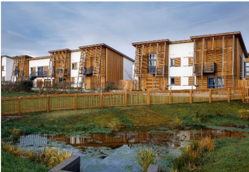
Figure 91 - Hanham Hall, South Gloucestershire: 187 homes built from factory made elements which minimise waste and are energy efficient to produce and build, the zero-carbon standard is achieved by using an efficient building envelope constructed using Structural Insulated Panels (SIPs) and roof-mounted PVs. The homes combine stack and cross ventilation, large openings, deep roof overhangs, balconies and shutters to avoid overheating.
