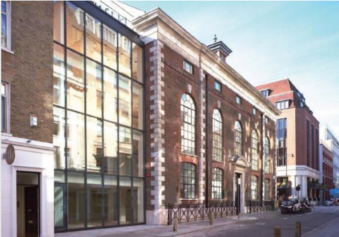
Figure 98 - Wren House, Hatton Garden: Originally built as a church in c.1670, it was then adapted for use as a charity school in 1696, before being reconstructed internally to provide contemporary office space. The original Grade II listed facade has been restored and retained.
