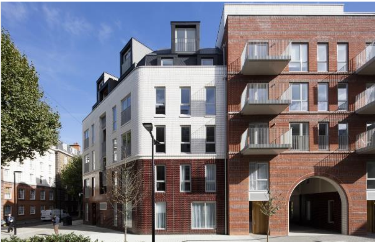
Figure 8 - The Bourne Estate, Camden: A sensitive contextual approach introduces two new blocks within an existing Grade II listed estate to complete the original layout. The buildings respond to the form and scale of the original architecture with fine brick detailing and a high-quality finish.
